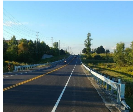
Figure 2.3: Paved Shoulder Example
