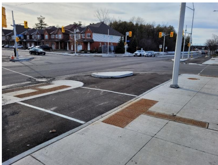
Figure 4.5: Directional TWSI at a Protected Intersection (Ottawa)
